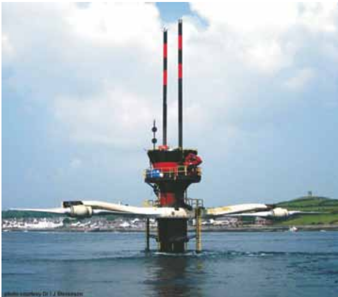
SeaGen in Strangford Lough with its rotors raised
